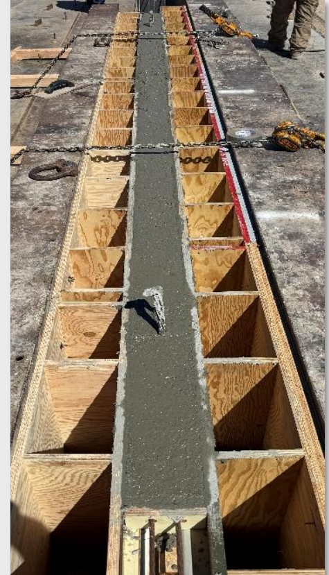
Figure 20: Finished Pour
