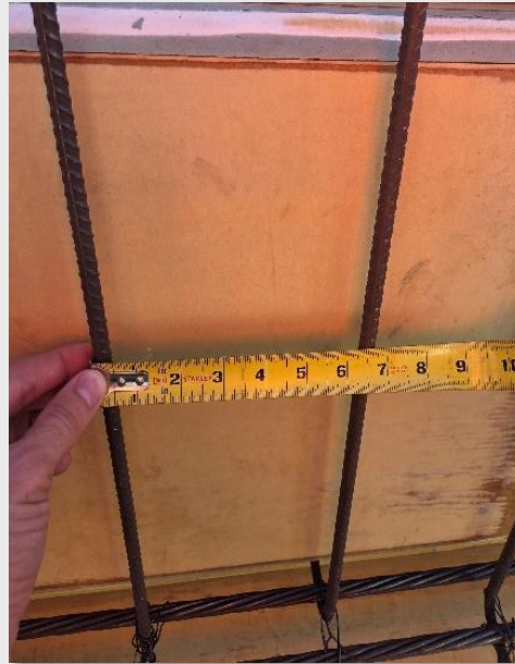
Figure 11: Verification of 6.50 in. Stirrups
