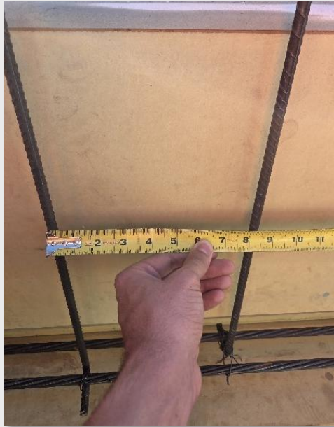
Figure 10: Verification of 8.25 in. Stirrups
