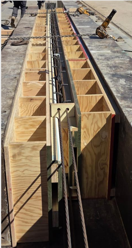
Figure 16: Beam Formwork
