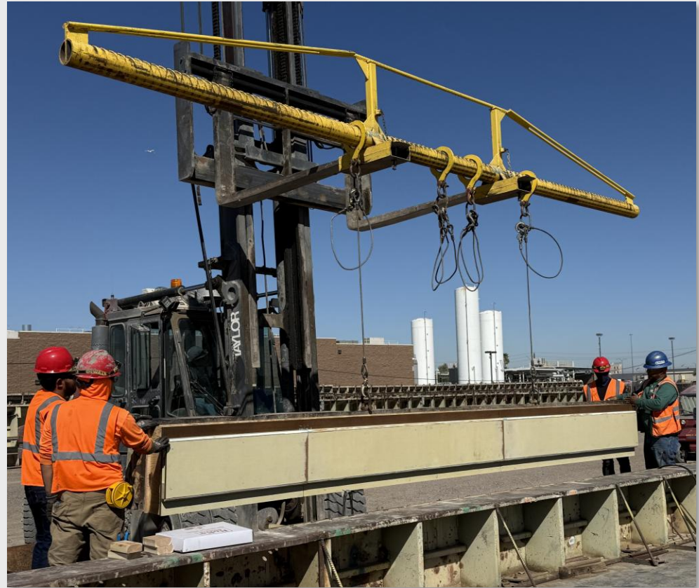
Figure 17: Tpac Workers Placing Formwork Together
