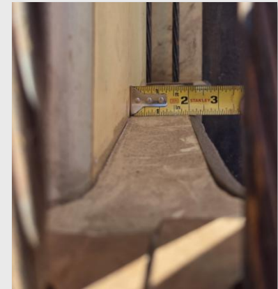
Figure 13: Verification of Web Thickness
